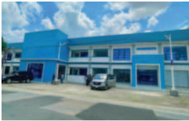
TRAINING HUB. TESDA's Provincial Training Center in Barangay Crispina, Banna, Ilocos Norte, following its launch on March 24, 2026. TESDA Secretary Kiko Benitez told senators on Tuesday (Sept. 15) that the country risks losing its demographic advantage if it fails to expand access to technical-vocational education. (PNA photo by Leilanie Adriano)
