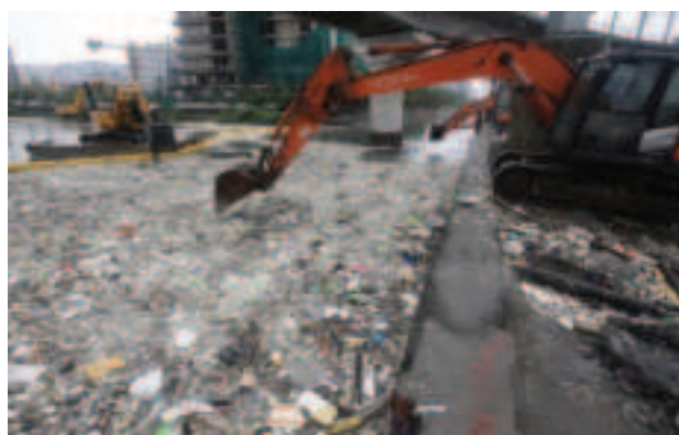
LONG-TERM SOLUTIONS. An excavator clears tons of garbage that washed into the Redemptorist Water Channel in Baclaran, Parañaque City on Aug. 12, 2026. The Department of Environment and Natural Resources on Friday (Aug. 13) pushed for long-term solutions to address the country's garbage problem. (PNA photo by Avito Dalan)
