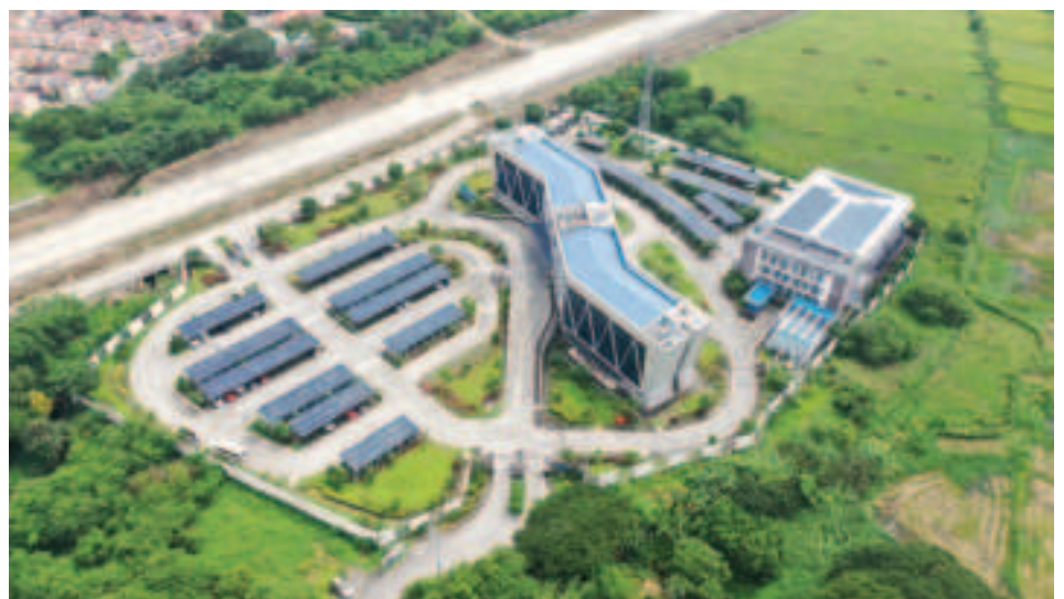
Aerial view of the MPT South Hub, featuring 1,184 solar panels that generate about 97% of the building's energy needs. The facility also has a rainwater harvesting system that reduces water use by 10%, along with EV charging stations for company electric vehicles.
