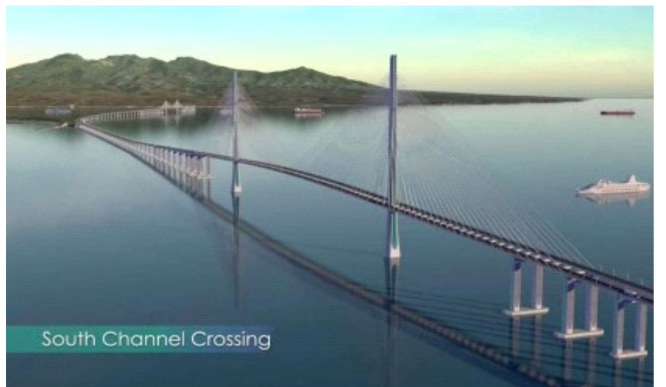
Bataan-Cavite Interlink Bridge (DPWH photo)
