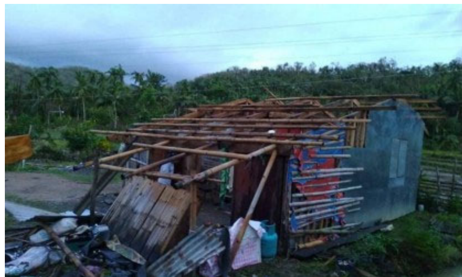
QUINTA'S WRATH. A house made of light materials was destroyed in the aftermath of Typhoon “Quinta” in Bato, Catanduanes on Tuesday (Oct. 27, 2020). The NDRRMC has estimated the typhoon's cost of damage to agriculture and infrastructure at around PHP429 million. (Photo courtesy of Radyo Pilipinas Catanduanes)
