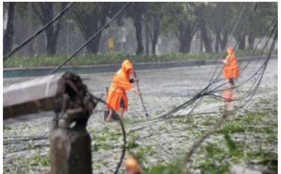
POWER OUTAGE. Electrical wires along Padre Burgos Street in Manila are damaged by Tropical Storm Enteng on Monday (Sept. 2, 2024). Meralco said 4,000 customers, mostly in Metro Manila, Cavite, and Rizal, were experiencing power interruptions on Tuesday (Sept. 3, 2024) due to the impact of inclement weather. (PNA photo by Yancy Lim)
