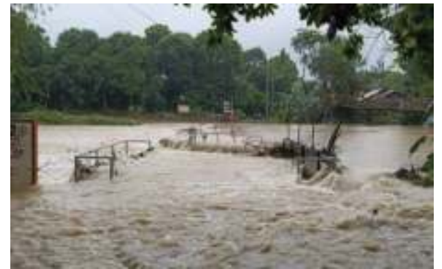
FLASH FLOOD. A spillway is flooded in Pozorrubio town, Pangasinan on July 25, 2024. Rizal Commercial Banking Corporation chief economist Michael Ricafort on Monday (July 29, 2024) said a 25 basis points (bps) interest rate cut next month is still possible despite the projected slight hike in consumer prices due to the effects of Super Typhoon Carina and enhanced southwest monsoon. (Photo courtesy of Pozorrubio Councilor Dennis Uy's Facebook account)
